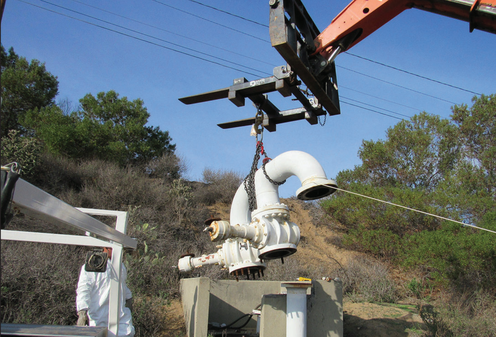
Closure contractors remove the 14-inch JP-5 cross connect valves at DFSP San Pedro. Photo by Carl Lind
