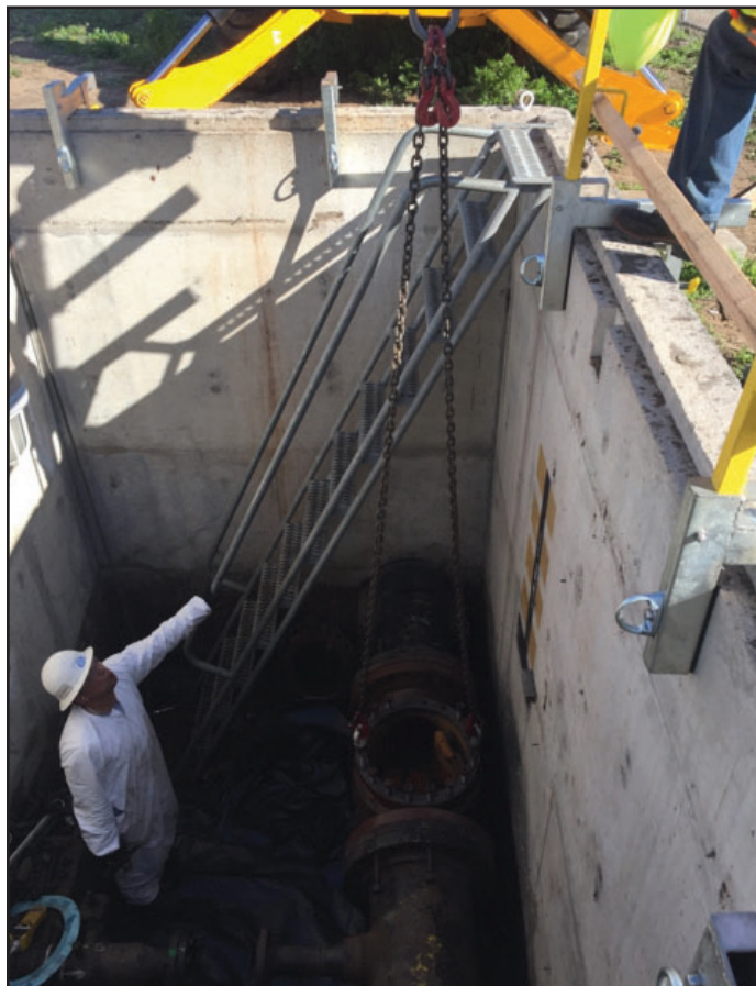
Closure contractor personnel remove an 18-inch double block and bleed valve south line stop valve from DFSP San Pedro’s Valve Pit 91. Photo by Carl Lind
