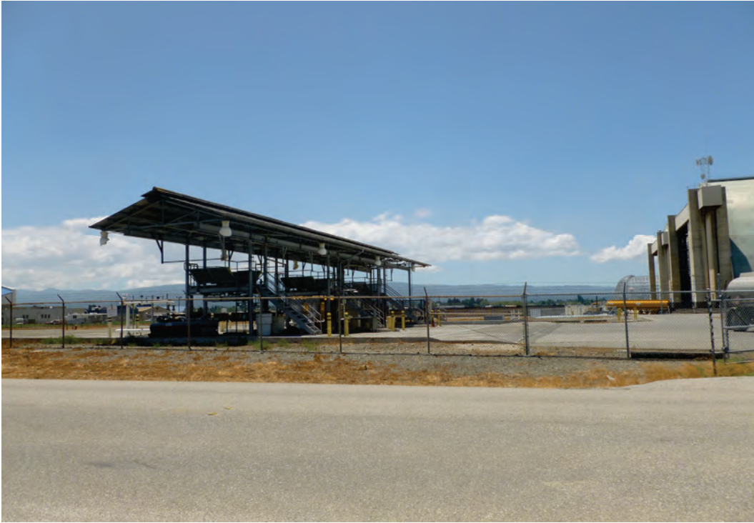
Plate 9. Building 141, view facing west
