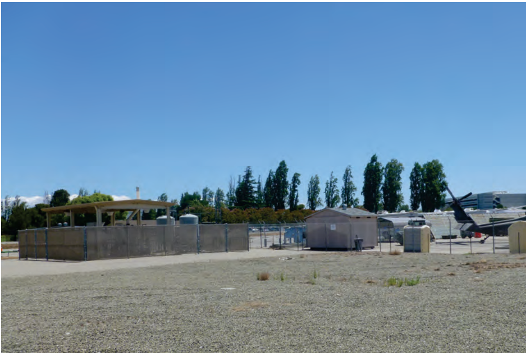
Plate 5. Building 439, at left, view facing southeast
