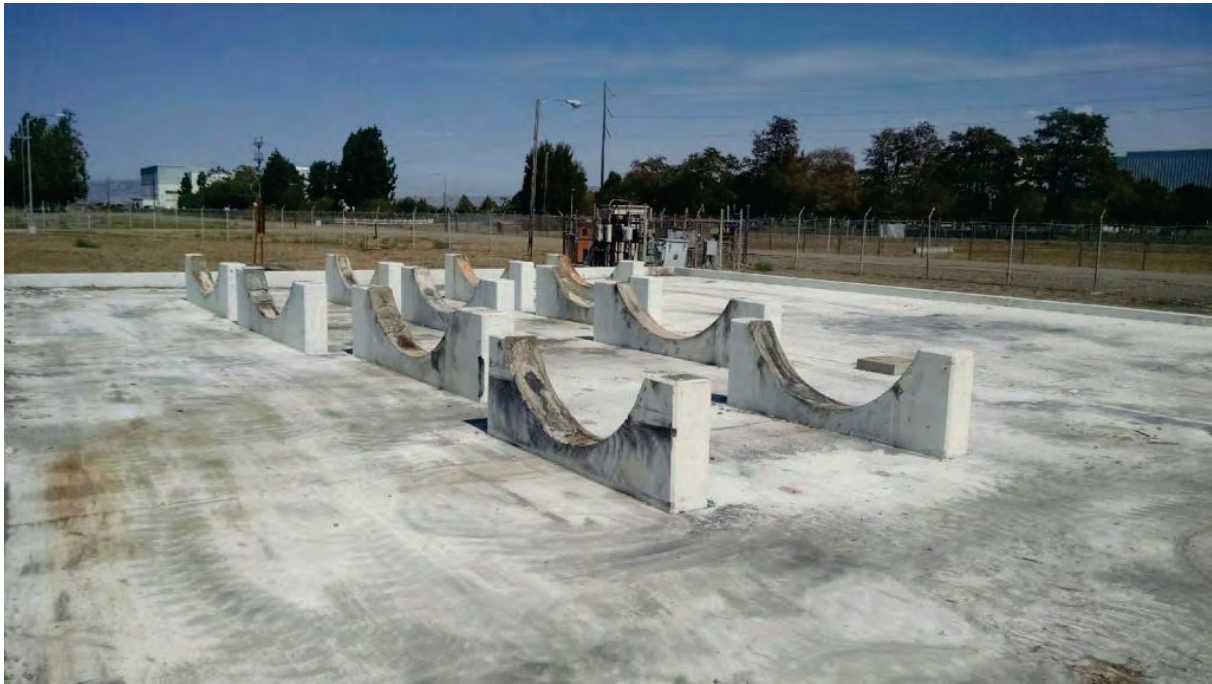
Fuel Farm after Removal of Aboveground Storage Tanks
