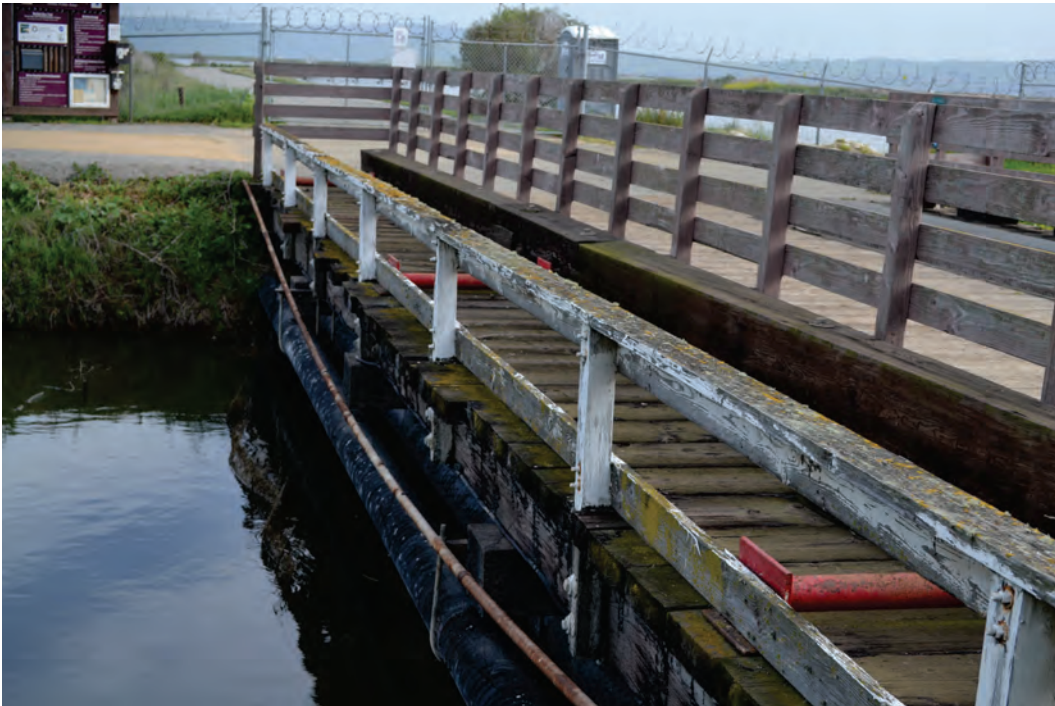
Plate 10. Building 169 (Bridge), view facing northeast
