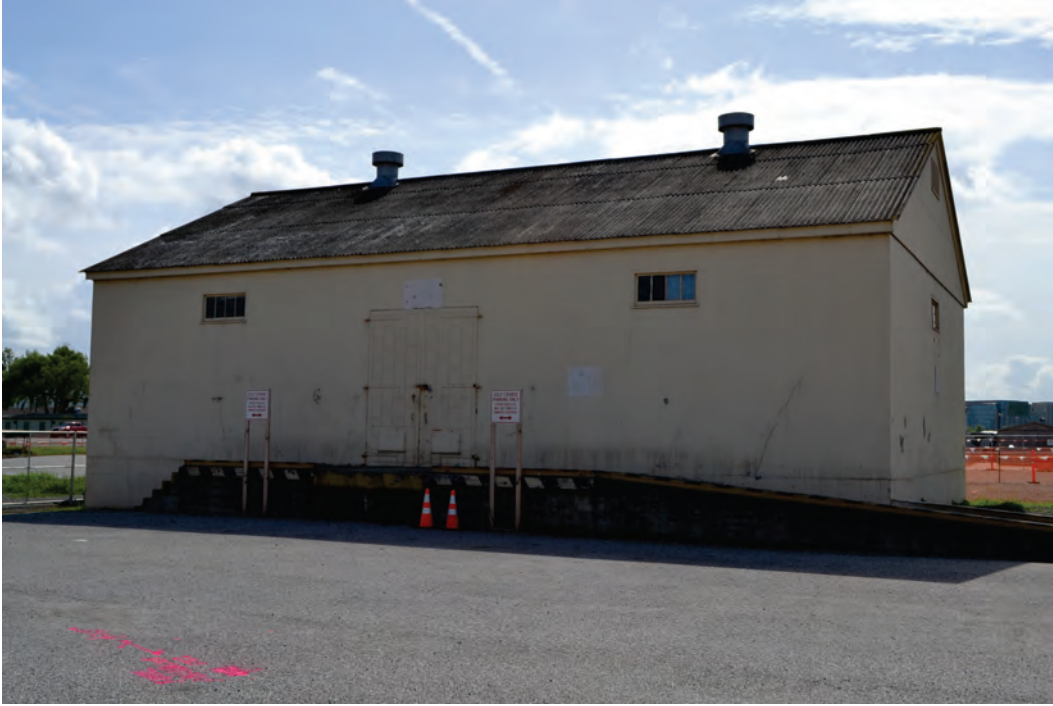
Plate 4. Building 69, view facing southeast
