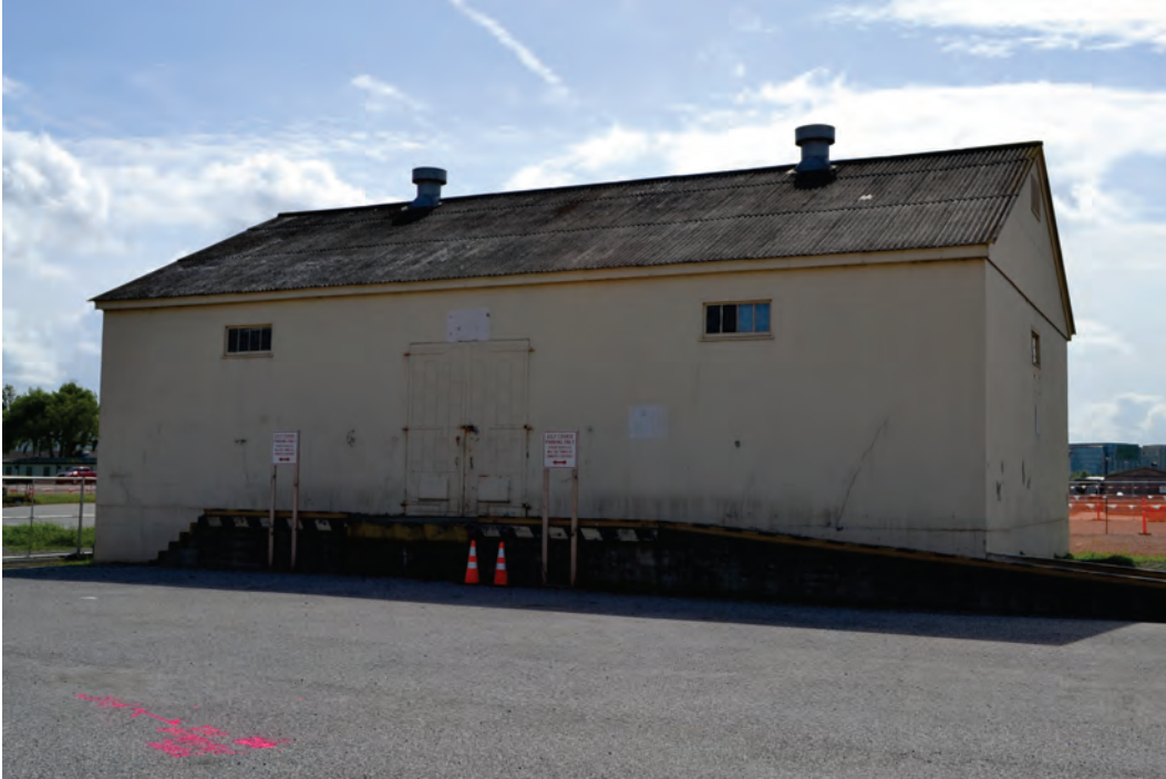
Plate 4. Building 69, view facing southeast
