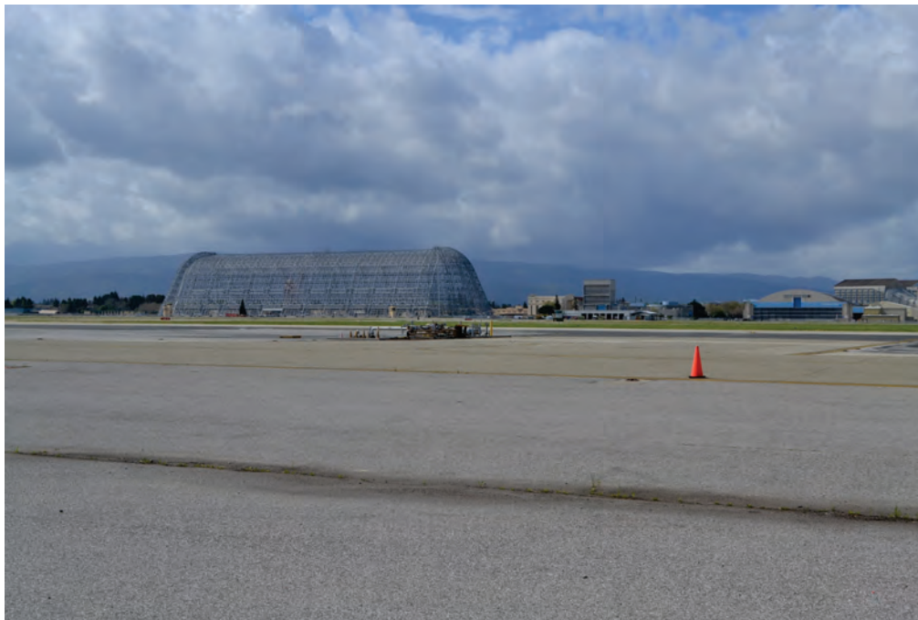
Plate 7. MF1016, taxiway pavement, view facing southwest
