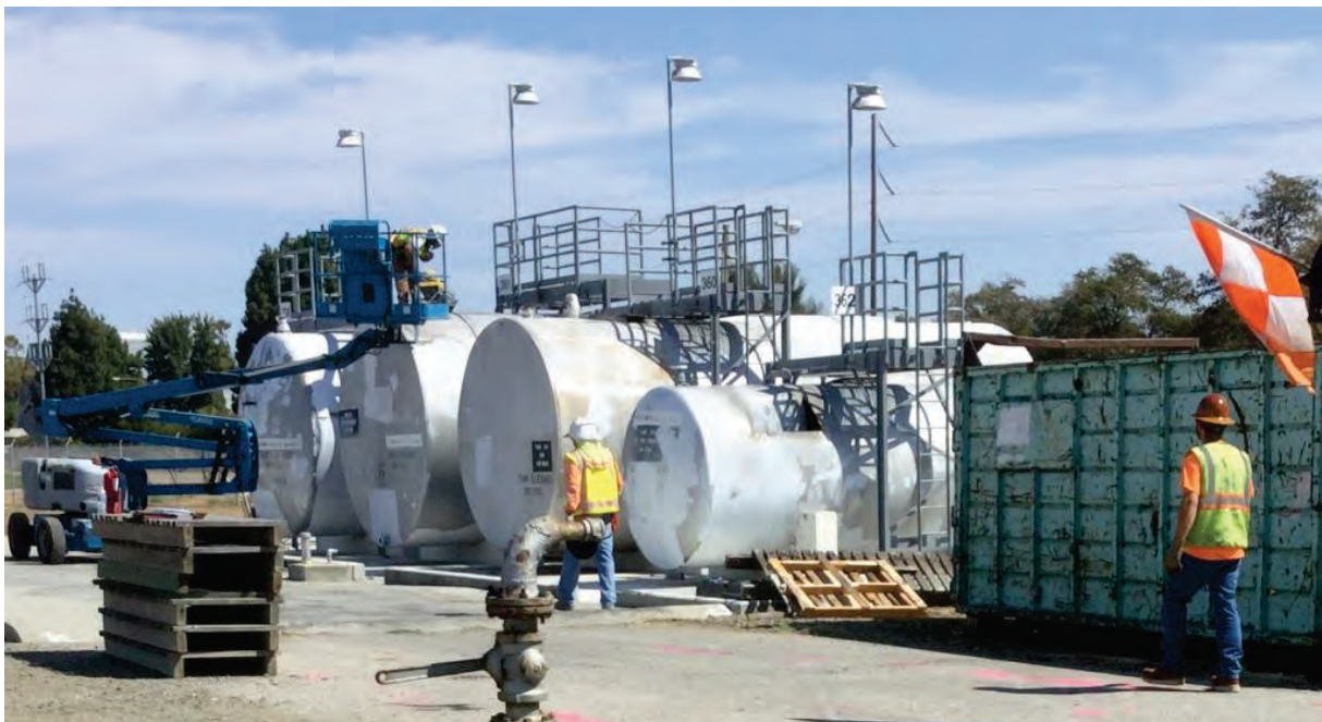
Crews Cutting Plumbing and Catwalks from Aboveground Storage Tanks
