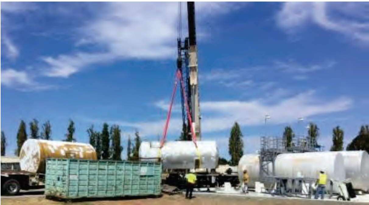
Crane Hoisting Aboveground Storage Tanks onto Flatbed Trucks
