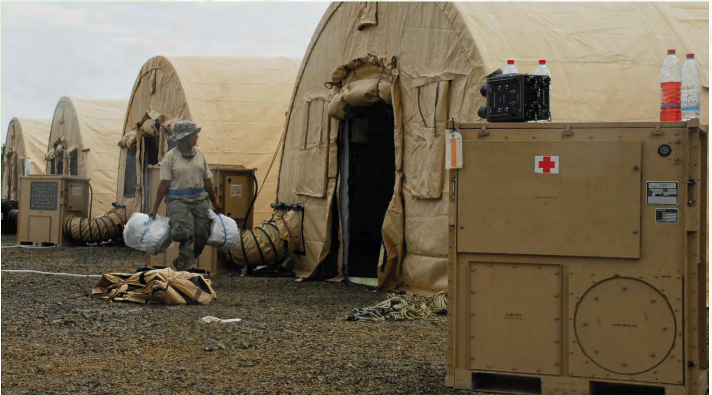
Airmen assigned to the 633rd Medical Group begin construction on the Monrovia Medical Unit site in Monrovia, Liberia. DLA provided building materials such as plumbing and electrical gear, lumber and fencing.
