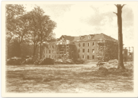
1942 image of construction on the Depot
