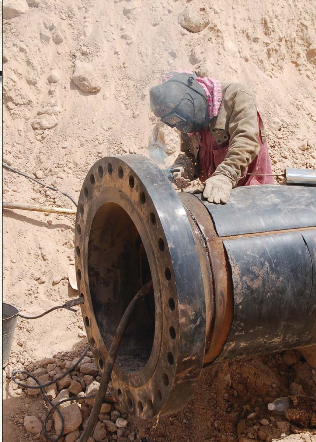
An Iraqi welder works in the desert heat to repair a severed oil pipeline in northern Iraq July 10, 2007. During the mission to restore Iraq's oil infrastructure, insurgency was on the rise and pipelines were often blown up in an attempt to delay the U.S. military's progress. Photo by Army Maj. Juanita Chang
