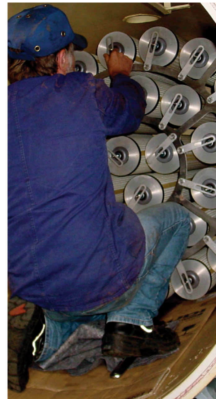
A workman changes worn out filters on the high pressure microfilter at the Pfungstadt depot along the Central European Pipeline System. The filter cleans sediment out of the petroleum products transported through CEPS. Courtesy photo
