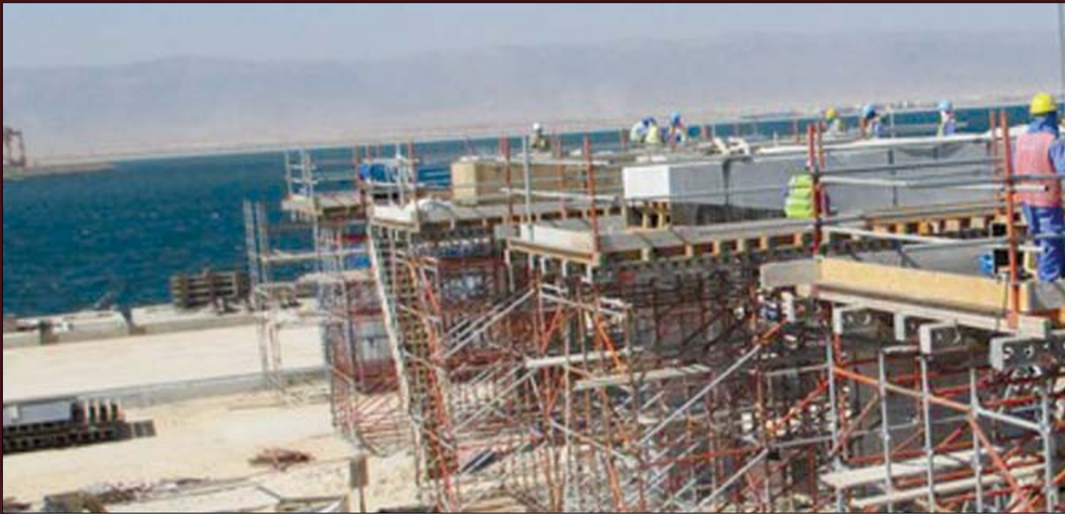
Workers work on crossover structure linking jetty pipeline to marine loading arms, a device consisting of articulated steel pipes that connect a tankship such as an oil tanker or chemical tanker to a cargo terminal. The construction is being done at a defense fuel support point in the Port of Salalah in Oman. Photo courtesy of DLA Energy Middle East.
