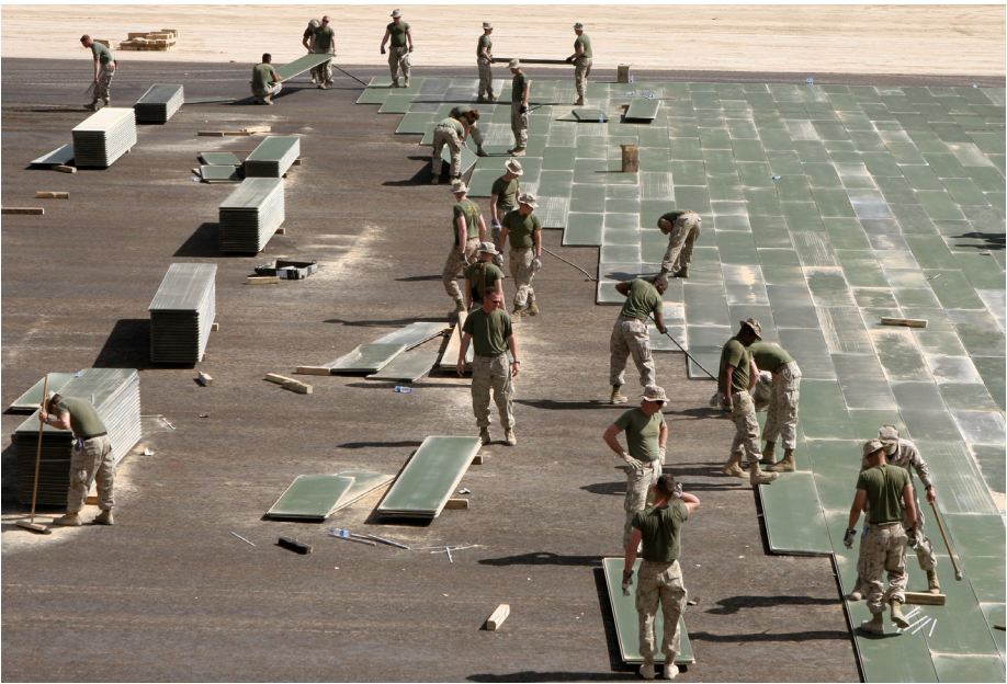
AM2 matting, shown here being laid down by marines from the 24th Marine Expeditionary Unit, allowed C-17 Globemaster IIIs to deliver mine-resistant, ambush-protected vehicles to southern Kandahar Province, where Cpl. Andrew Carlson took this photograph in March 2008. DLA provided this matting either directly or through the Air Force.
