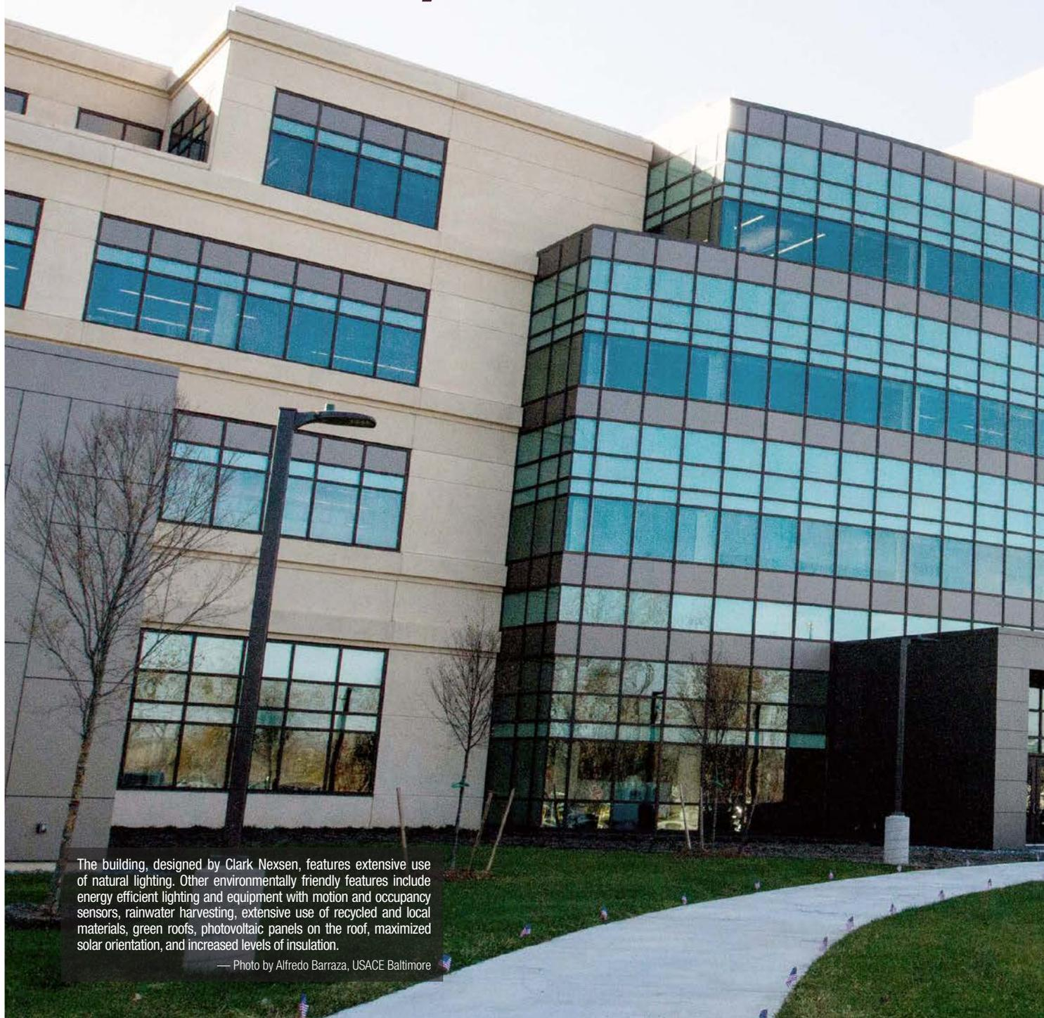
The building, designed by Clark Nexsen, features extensive use of natural lighting. Other environmentally friendly features include energy efficient lighting and equipment with motion and occupancy sensors, rainwater harvesting, extensive use of recycled and local materials, green roofs, photovoltaic panels on the roof, maximized solar orientation, and increased levels of insulation.
