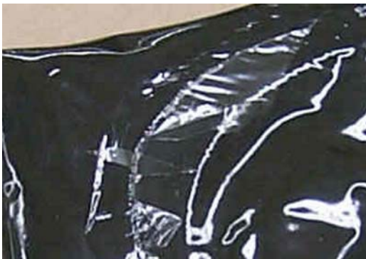
Outer- Ply Delamination - Propagated
